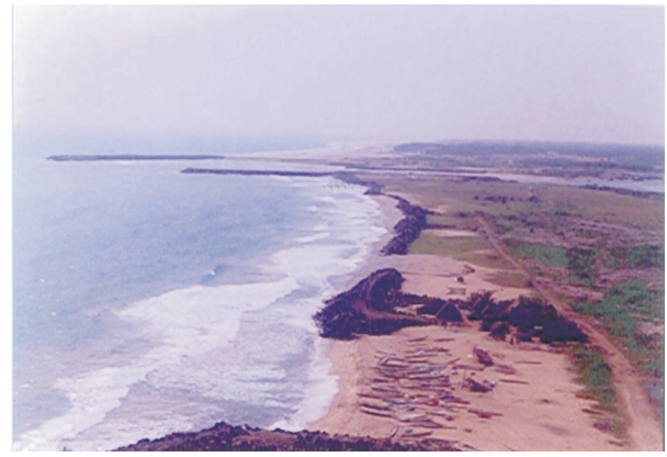
Figure3. View of the Pondicherry Harbor (See the accretion of sand at the far end of the photo).
